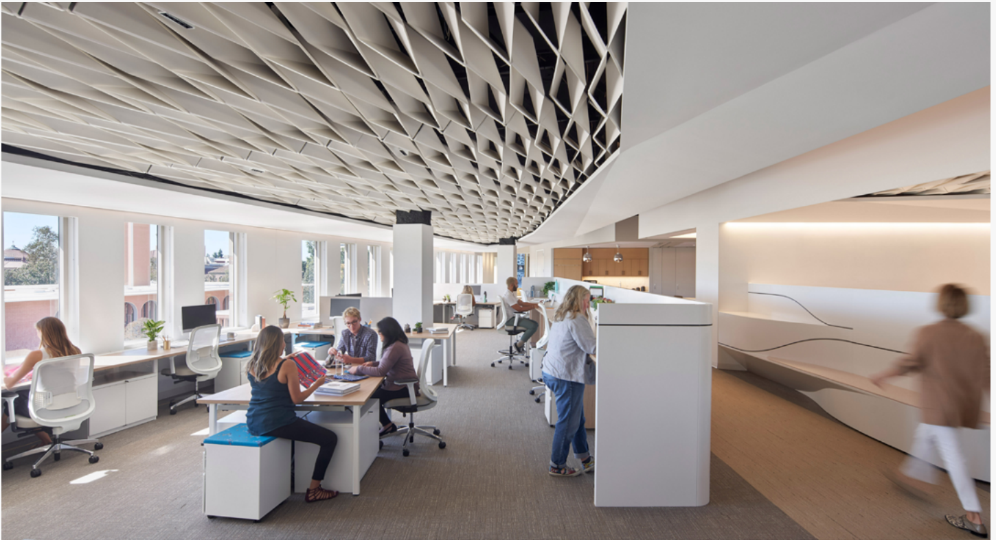
Faceted Acoustic Ceiling Feature
